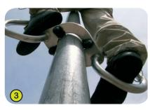
3- The climbing system (feet) is made of stainless steel.
