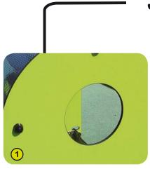
1- The coloured panels are made from a 13mm thick compact material (HPL). Robust in construction, it offers excellent resistance to weathering and vandalism.
