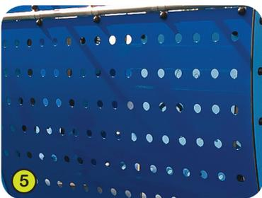
5- **The cabin** is made of 3mm thick perforated aluminium coated with polyester epoxy lacquer.
